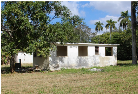
Figure 5. General view of the GNSS service building from the south side.
