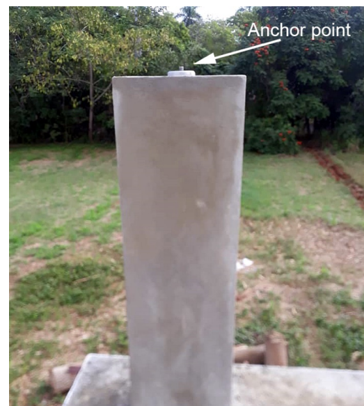
Figure 7. Concrete pillar with a platform for a GNSS antenna mounting.
